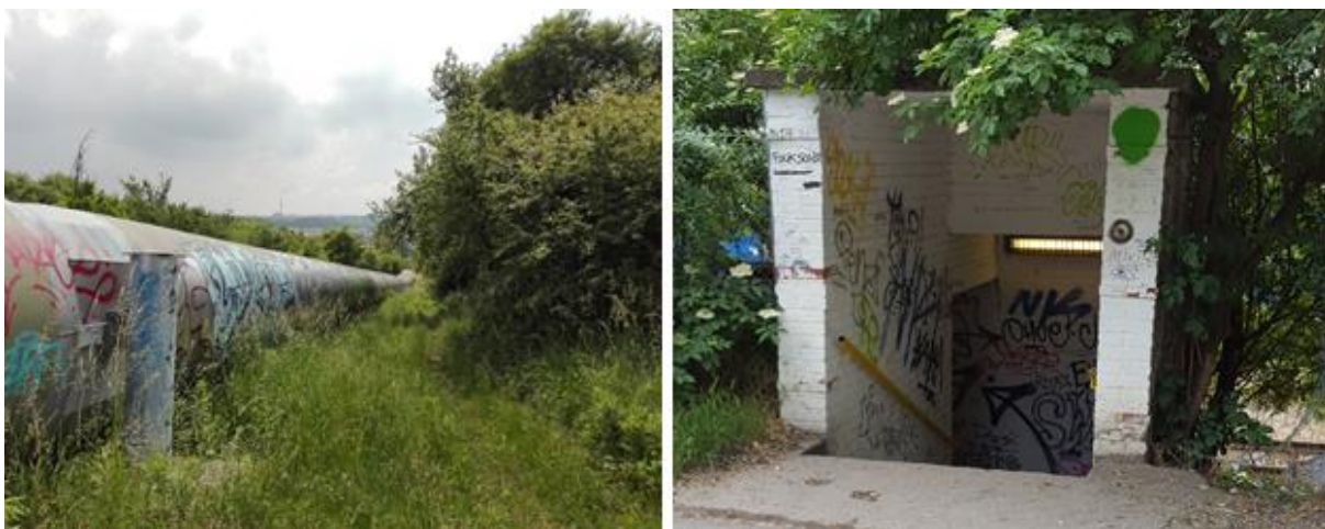
Figure 6. (Left) heat transportation pipe in the east part of Vysočany Hill, (Right) one of the pedestrian tunnels under the train tracks
